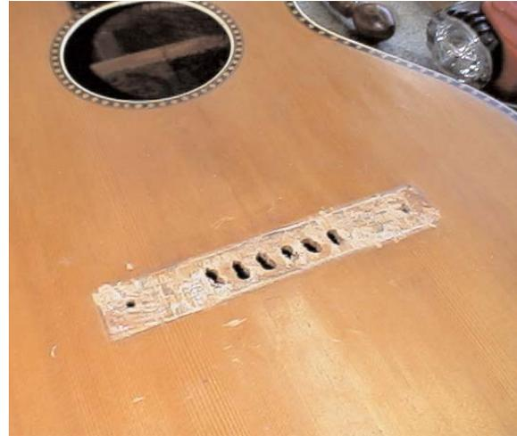
The next day, Day 2, I took my inspection mirror to see how the bridge was bolted on. What I noticed was the bridge plate had been partially cut and removed, further weakening the top. I assume the partial removal was to help the top vibrate more for a “better” sound and was done when the top and/or back was removed. It couldn’t have been done any other way. After inspecting, I then proceeded to remove the old bridge.
