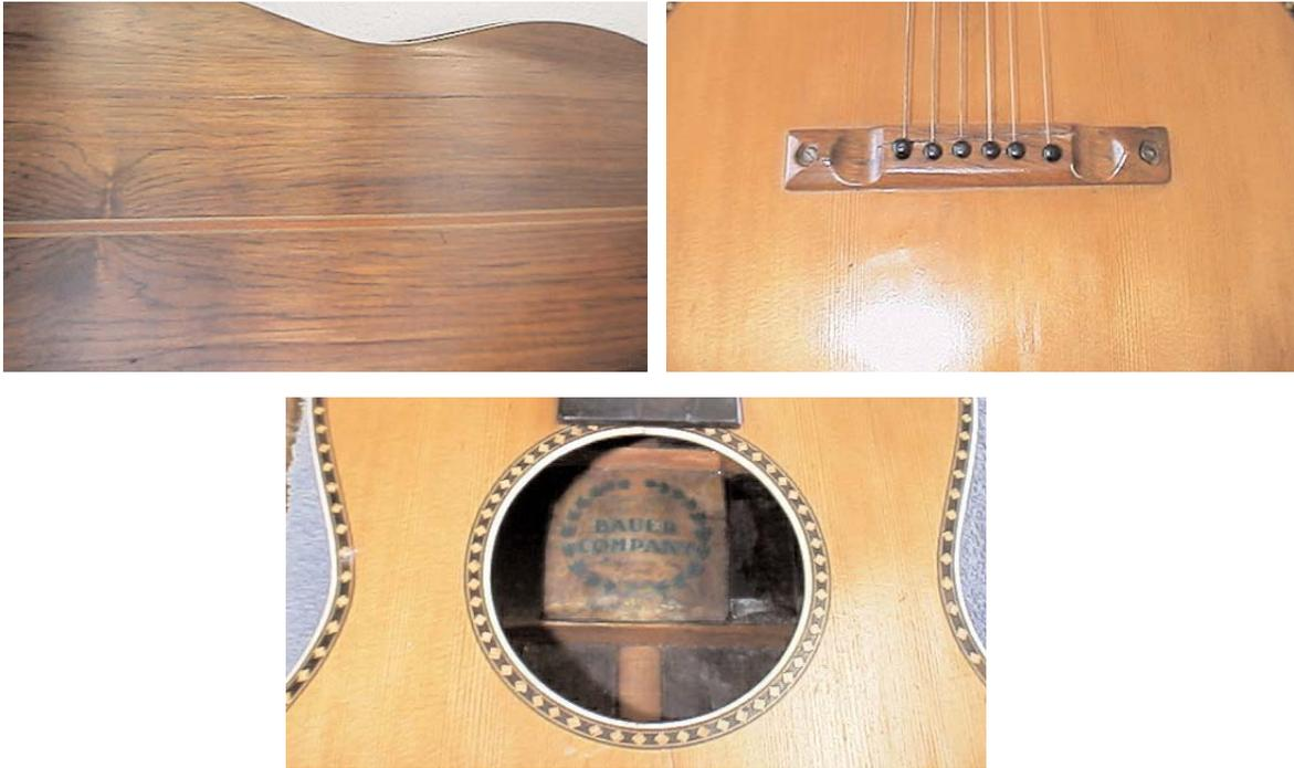
On Day 1, I conducted a more extensive assessment of needed repairs and came up with some interesting findings. I noticed that the back cracks were caused from loose back braces, so there was not much support for the thin rosewood back. I would have to fix the braces before I could repair the cracks.
